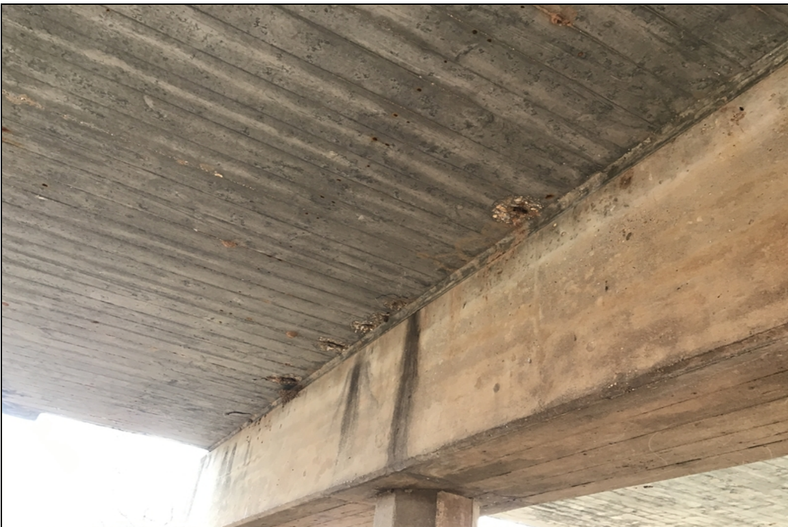
Soffit - Span 2 @ Bent 3 left: Rebar exposed
