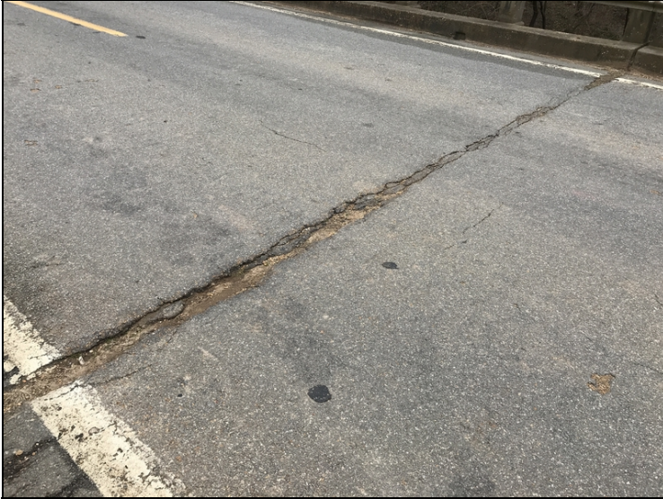
Wearing surface - Bent 5: Deterioration (potholes)
