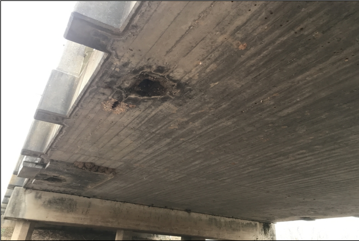
Soffit - Span 2 right: Patched/spalling
